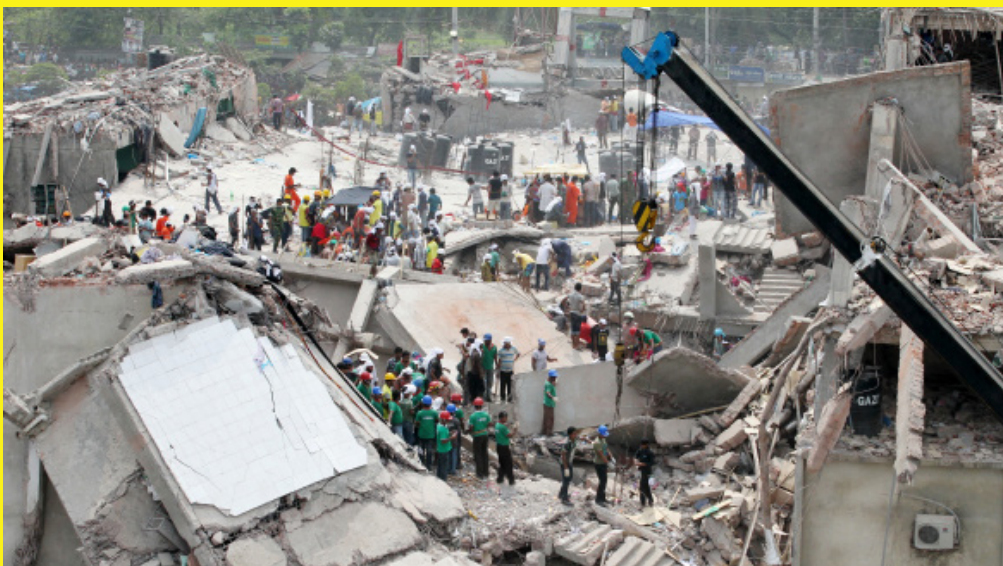
← The aftermath of the Rana Plaza collapse. Photo by Shutterstock / Bayazid Akter.
